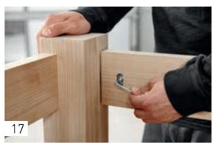
Tighten the connection using a 4 mm hexagonal socket.
