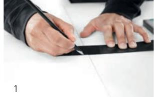
Mark out the connector position on the surface of the worktop at the desired point. Also mark the positions for additional dominos (used to ensure a flush connection).
