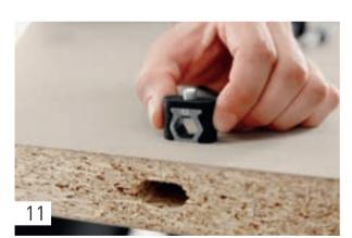
Insert the transverse anchors into the routed holes.
