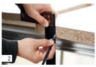
Transfer the markings to the abutting surfaces of the worktop. It is sufficient to do this where you later want to insert the flat connectors.
